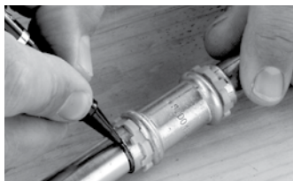
FIGURE 3: MARKING INSERTION DEPTH
